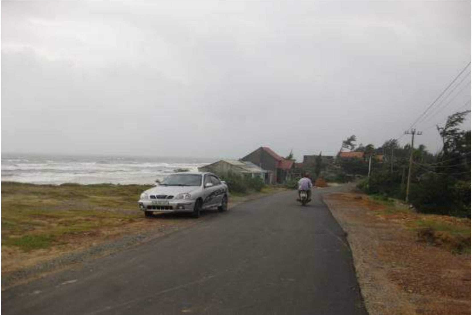
Road constructed over natural sand hills
